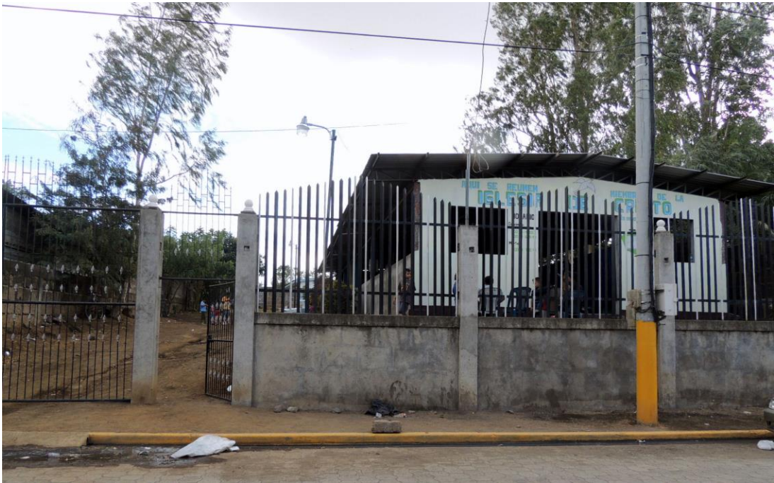
Tipitapa Centro church building
